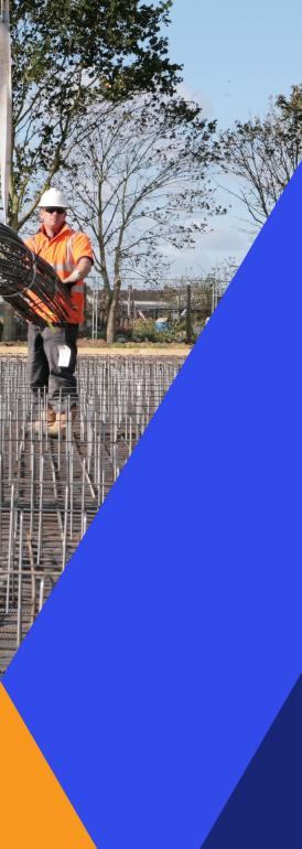
Comdeck is suited to almost all commercial projects and replaces the need for traditional strip foundations and pile and beam. It can cater for the required loads and building techniques of low to mid-rise structures. It is suitable for all types of construction, such as timber frame, sealed panels or modular. Adding hold down bolts and starter bars can also be incorporated within the slab design.
